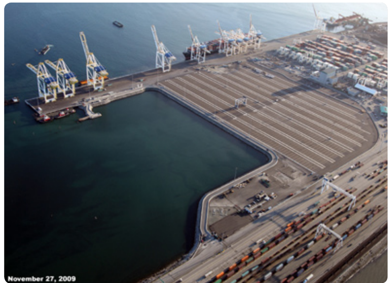
View of Deltaport Third Berth featuring TSI's three new 80LT quad-lift quay cranes.
