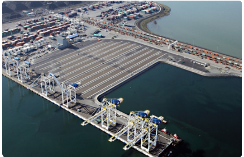
Deltaport Third Berth, showing progress on October 24.
