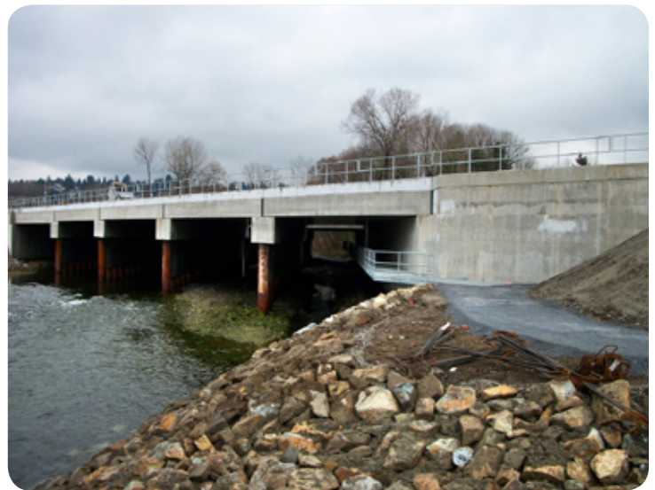
Lynn Creek Rail Bridge
