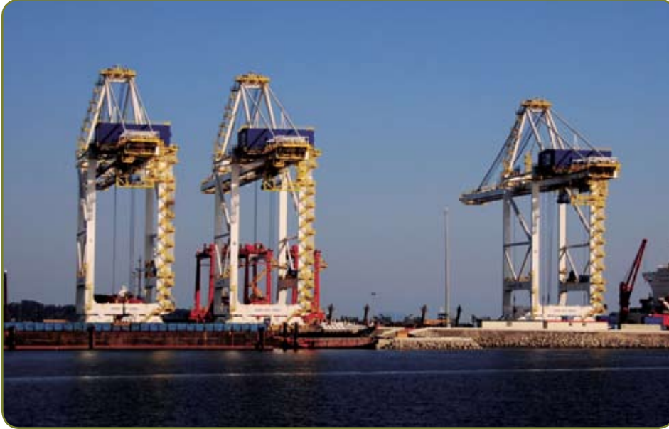
Deltaport container terminal received three new 80 Long Tonne (LT) Quad gantry cranes as part of the Deltaport Third Berth Project. Photo Credit: Jeff Edgar
