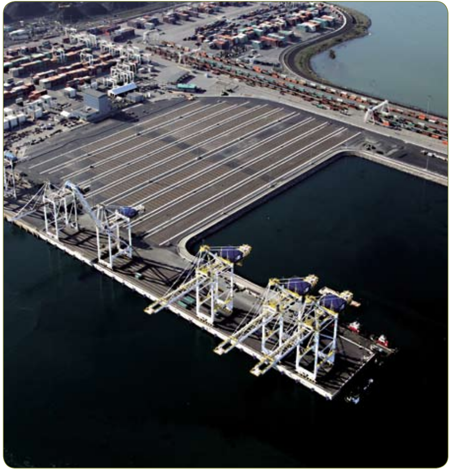
The Deltaport Third Berth, scheduled to open in January 2010, features three new Quad-lift gantry cranes. Photo credit: TSI Terminal Systems Inc.
